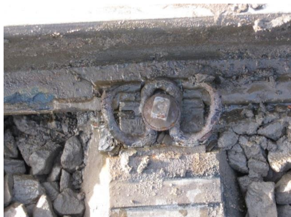
Fig.1. The corroded tension clamp at the level crossing. (full colour version available online)
